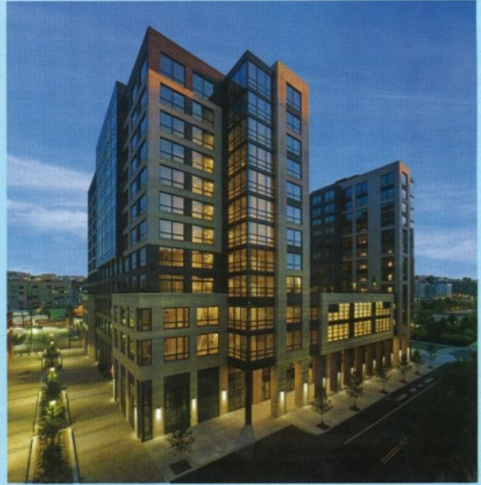
Park + Garden, a 212-unit rental project at 1450 Garden St. in Hoboken, was designed for LEED Gold certification when it opened in 2015.
